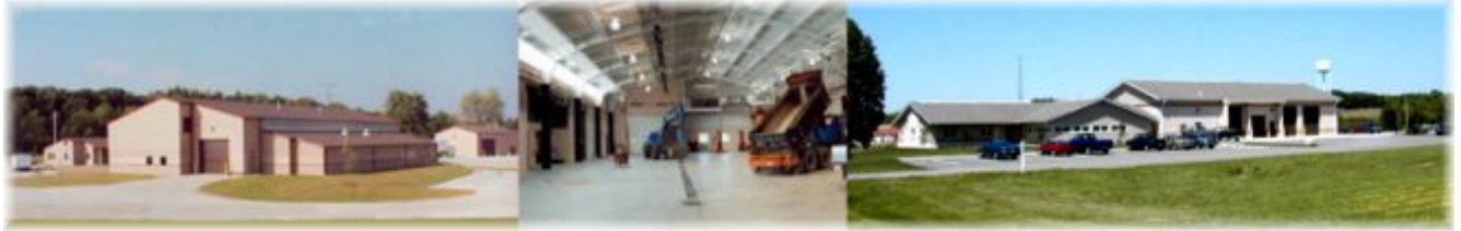
Pictured above on left, new county engineer's facility. At right, new water resources lab on Infirmiry Road
